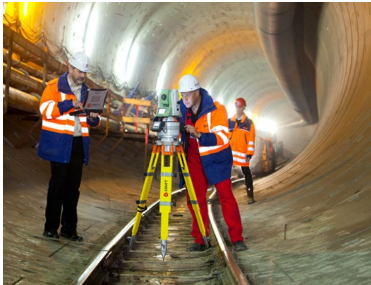
Tunnel survey with GYROMAT 3000
